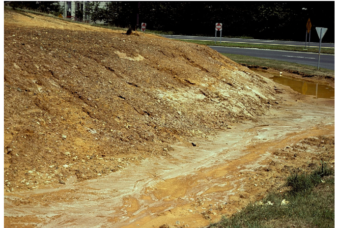
Construction site for ornamental flower meadow
